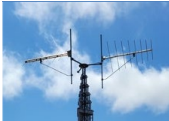
Figure 16. Back-to-Back, High Front-to-Back Ratio Antennas at FM2-FM3 Booster Site
