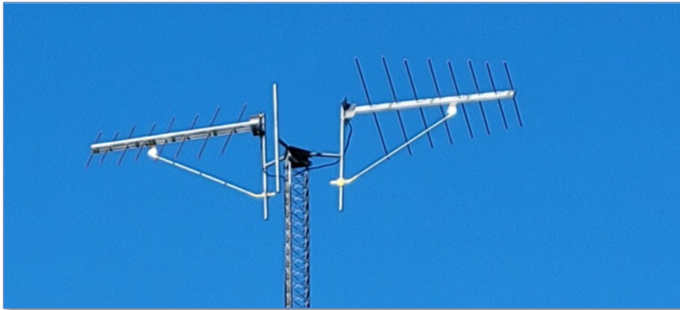
Figure 31. Back-to-Back Antennas at Highway 25 COW Site
